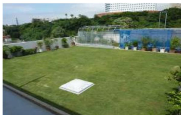
屋上緑化の推進 Promotion of roof greening
